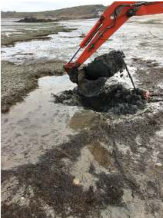
Plate 5.1 Mini digger being used to excavate old intertidal mooring block at Porthdinllaen (© National Trust/Laura Hughes)
