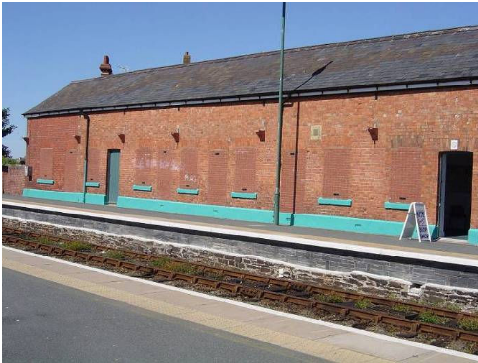
Tywyn Train Station before the work was installed
